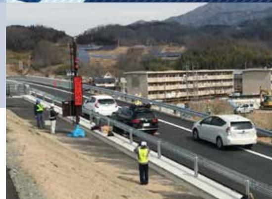
*A warning signalization system (e.g. a flashing beacon) along the exit ramp can be activated upon detection in order to warn the unsuspecting wrong-way driver about his or her mistake.*
